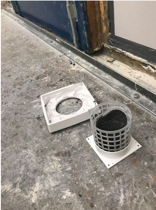
Picture 6 – The indoor part of the unit with dust and insect filter.
