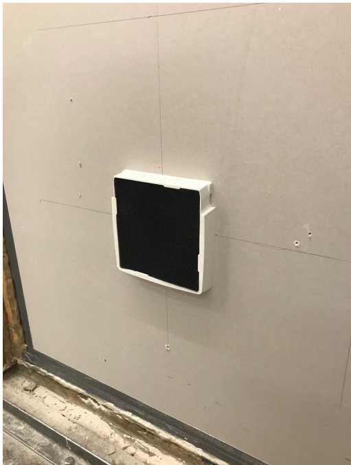
Picture 12 – The standard filter mounted.
