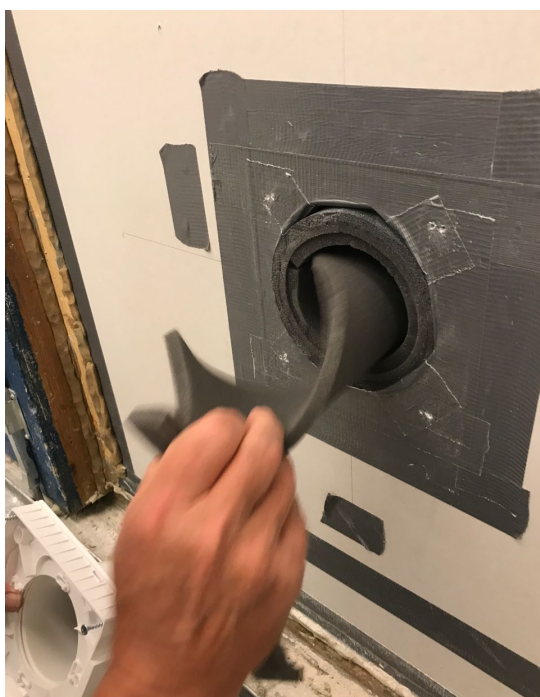
Picture 14 – The inner polyether foam ring was removed and replaced with an un-perforated filter cassette.
