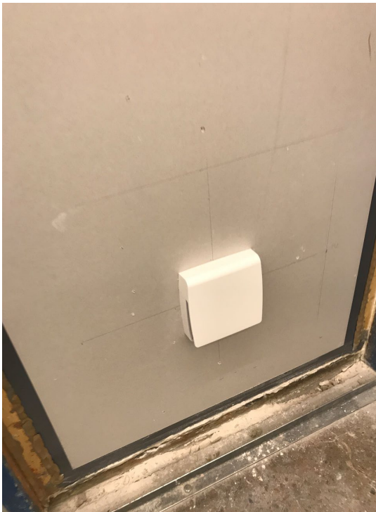
Picture 8 – The indoor unit mounted on the wall.
