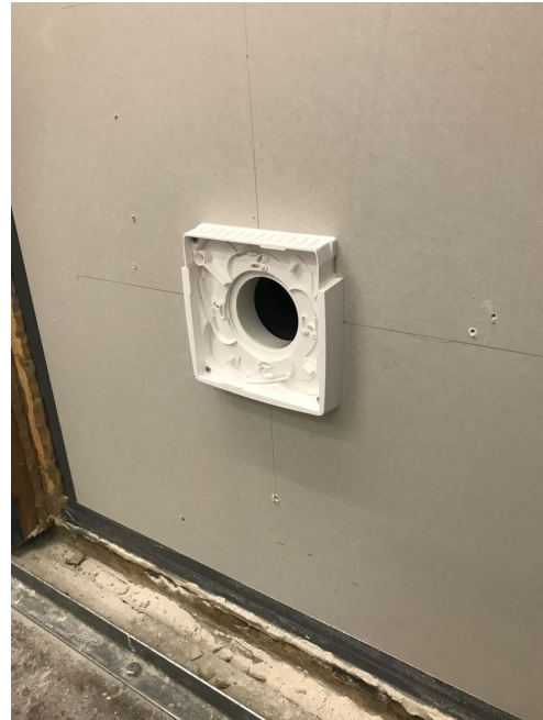
Picture 11 – The interior unit during assembly.
