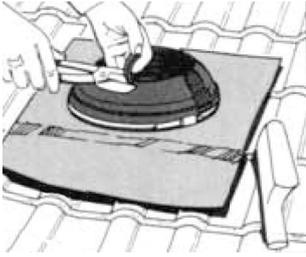
Trim the tile roof flashing cone to suit the tube size.
