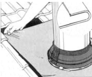
Flatten the sheet lead and form an anti-capillary fold (10mm x 2mm approx.).
