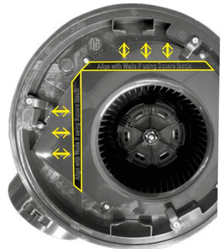
**Note: When installing with a square fascia, ensure it aligns with the walls. Refer to the interior marks on the EC Contour Fan for guidance.**
